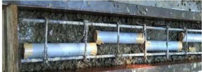
Fig.4: Casting of hollow beam
