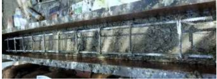
Fig.2: Casting of solid beam
