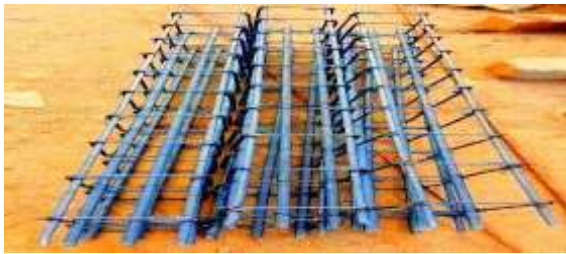
Fig.1: Reinforcement cage of control beam
