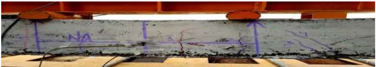
Fig.10: Crack Pattern of Hollow (40mm) beam
