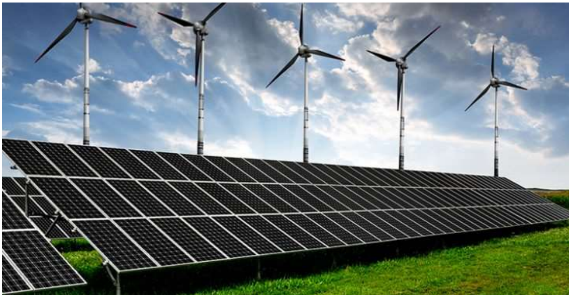
Figure 1.1: Hybrid Power Plant
